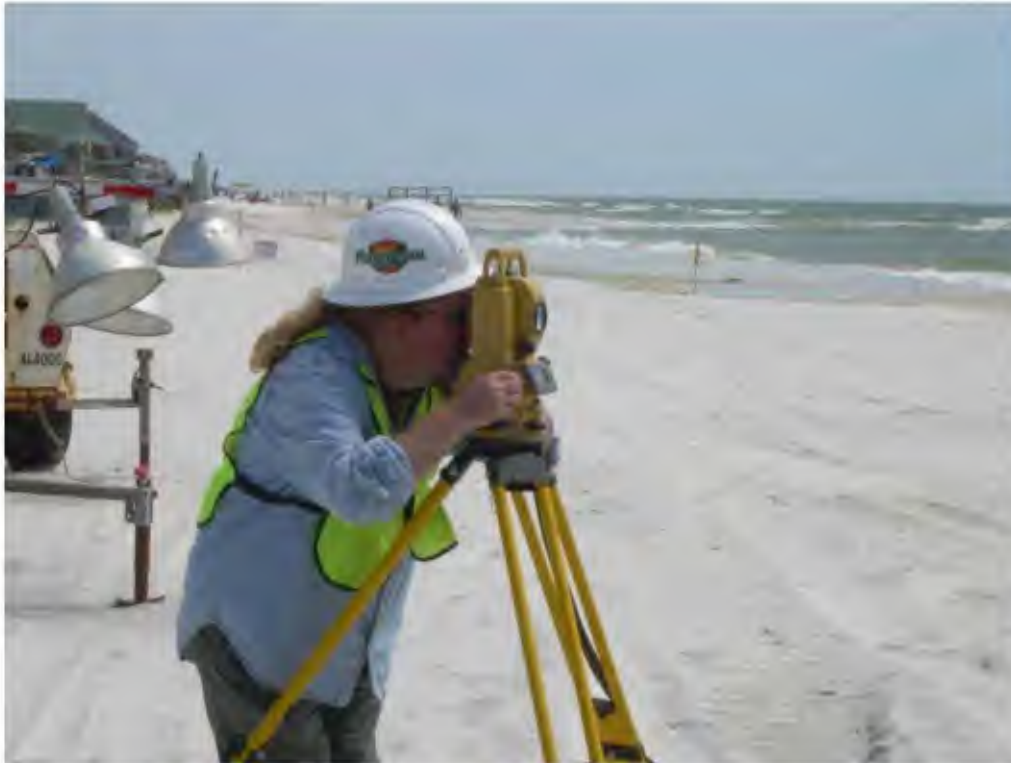
Figure 11-6. Total station control of topographic beach profiles.
